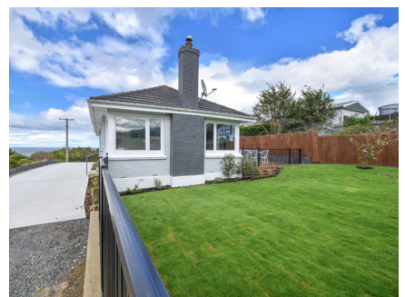
existing house after
